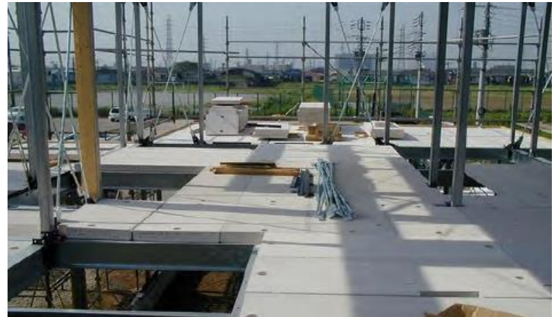
As Upper Floor Slab
