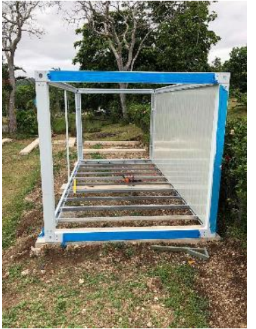
PBV System using light weight insulated wall panels can be designed as a 2 storey buildings and be fitted with En-suite prefab toilet module. The module can be lifted as one complete unit for relocation purposes
