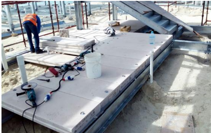
As Ground Floor Slab
