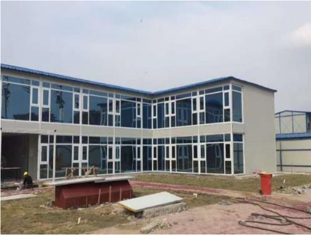
PBV System using light weight insulated wall panels can be designed as a 2 storey buildings and be fitted with En-suite prefab toilet module. The module can be lifted as one complete unit for relocation purposes
